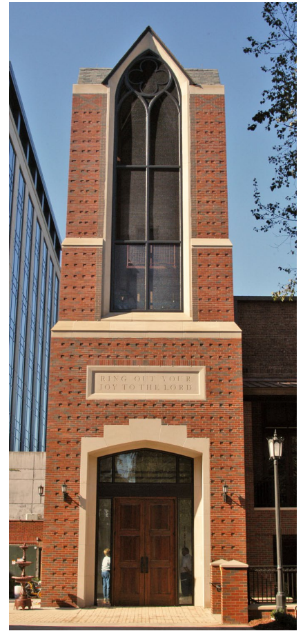
The finished tower
