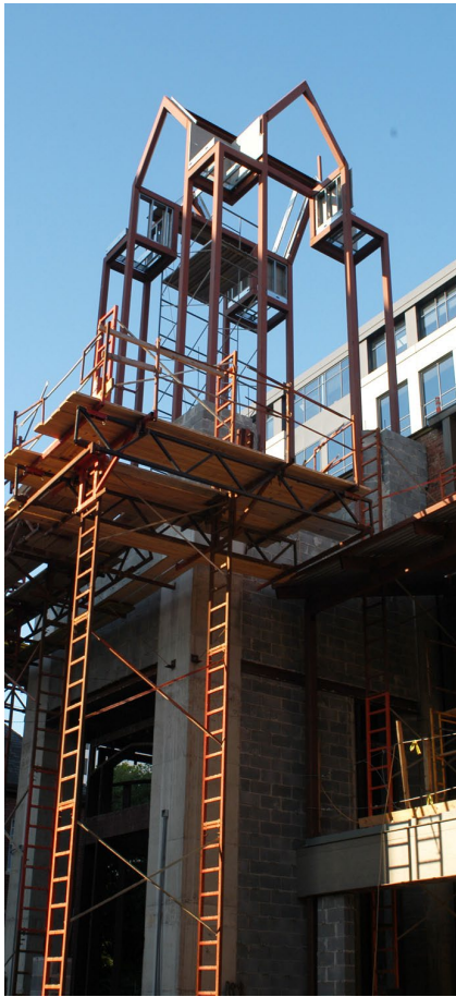
The tower under construction
