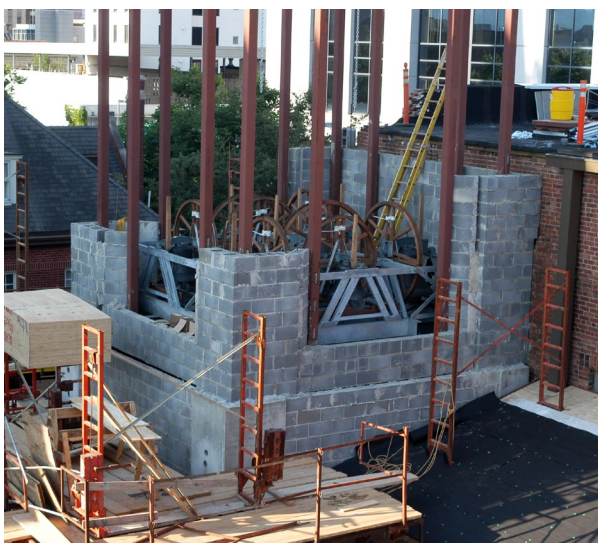
The bells installed in the unfinished tower
