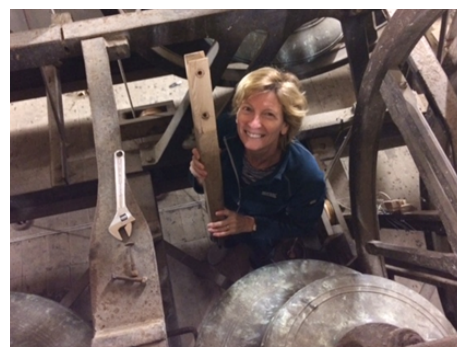
Lucy in the belfry, getting to grips with a cracked stay
